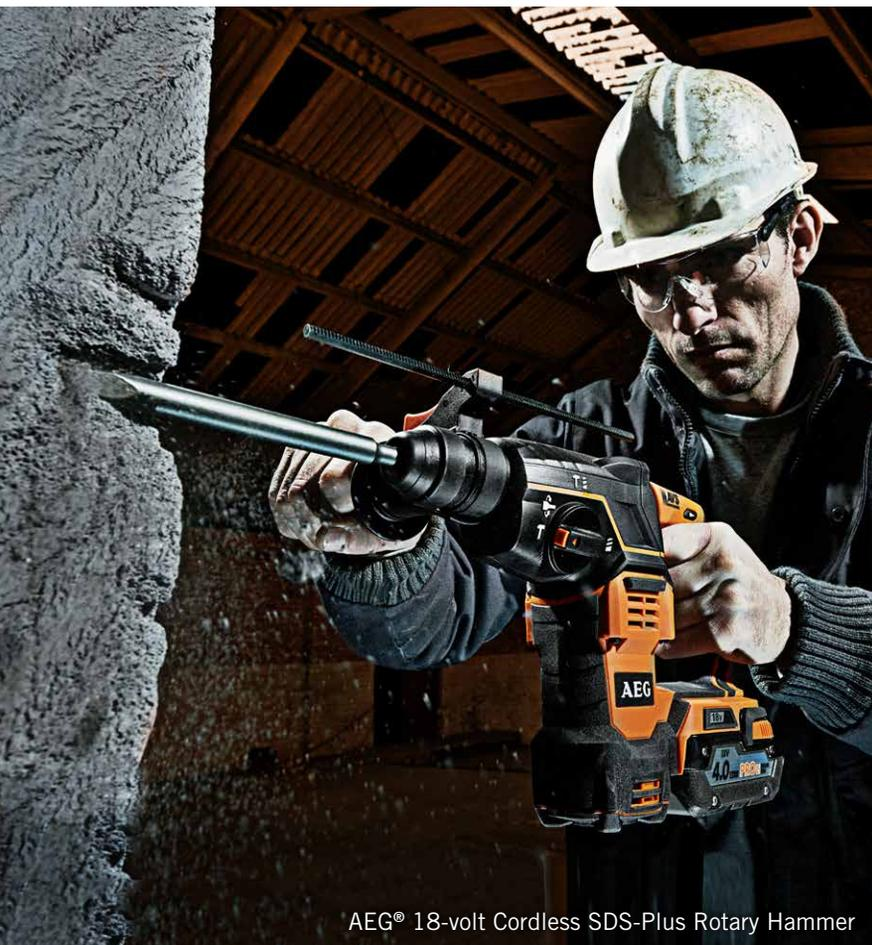
AEG® 18-volt Cordless SDS-Plus Rotary Hammer
